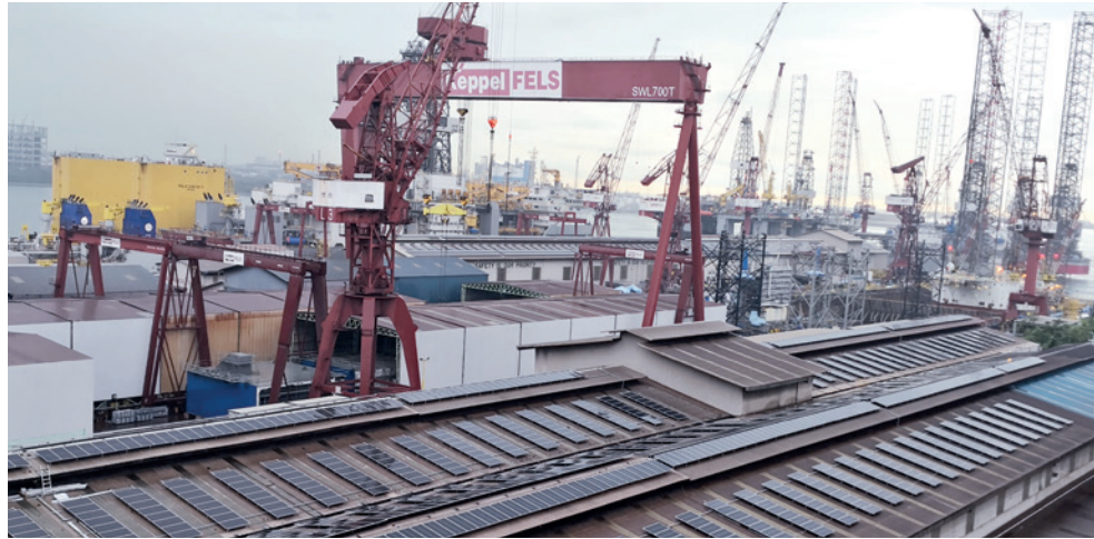
As part of its sustainability efforts, Keppel O&M installed 21,000 solar panels with a peak capacity of 8.8 MW at its yards in 2019 to offset its energy demand
